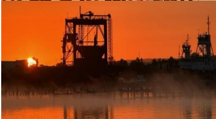
UE Local 106 Port Reading NJ. Buckeye pipeline
